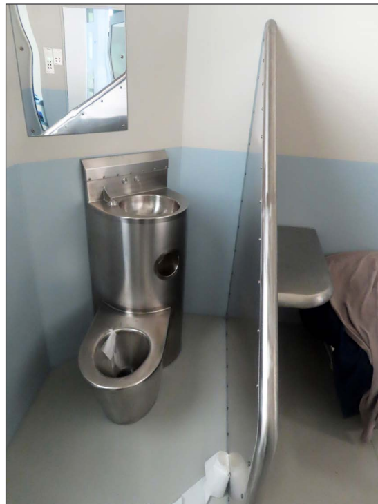
Photo 5: Integrated toilet in an accommodation room (Inspector of Detention Services staff removed from image)
