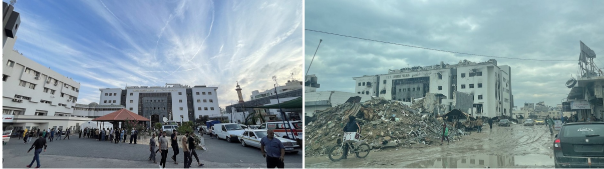
One building, one photographer. The special surgery building at Al-Shifa Medical Complex, Gaza City: on 11 October 2023, in the first week of the war (left), and on 23 February 2025, after two sieges (right). Photographs: Jaber Jihad Badwan, CC BY-SA 4.0, via Wikimedia Commons.
